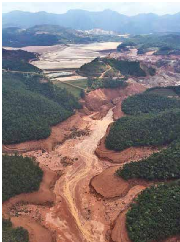
Figure 7 Devastation after the dam burst of the Samarco mine. Samarco dam failures via Estadão http://blogs.agu.org/landslideblog/2015/11/08/samarco-1/
