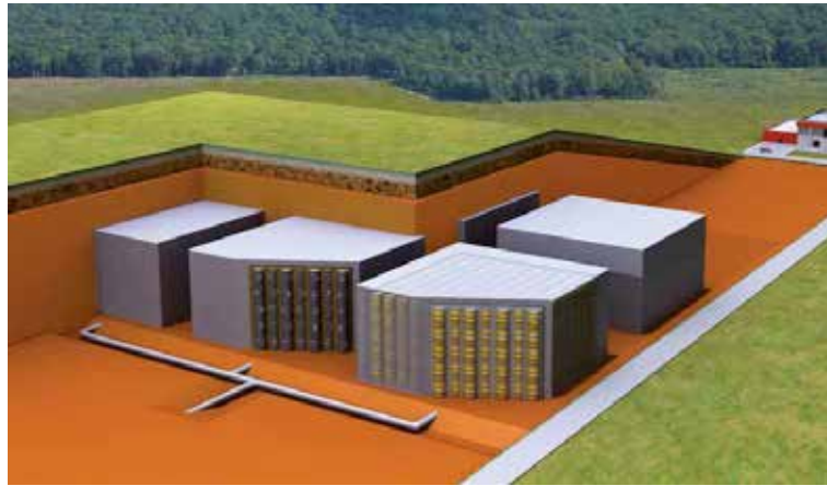
Figure 8 Concept of ANDRA of a surface disposal facility for ‘low- and intermediate-level short-lived’ waste. Source: [ANDRA-solutions 2014].
